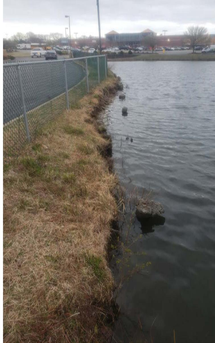
*An example of localized shoreline erosion in a retention basin.*
