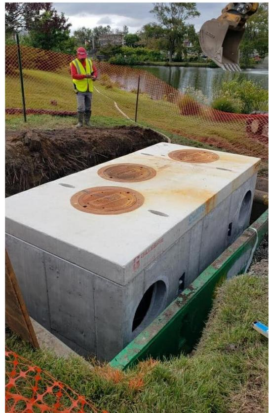
*An example of a manufactured treatment device during installation.*
